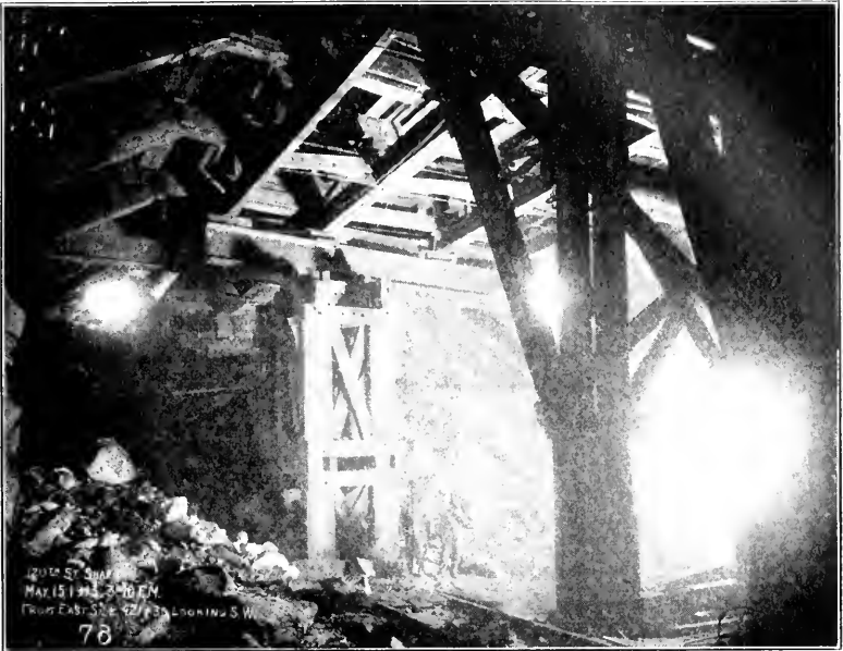
FIG. 14.—CONTINUOUS BEAMS, WITH CROSS-BRACING AND TURNBUCKLES.
